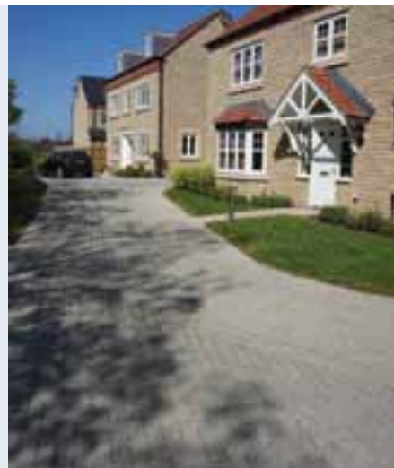
Bicester in Oxfordshire, is home to major new developments making extensive use of permeable, in conjunction with conventional, concrete block paving. Under construction now are Kingsmere (above) and the North West Bicester Eco-town.
