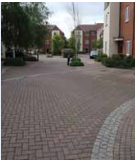
Concrete block permeable paving characterises this high-density town-centre housing project in Abingdon, Oxfordshire (above).
