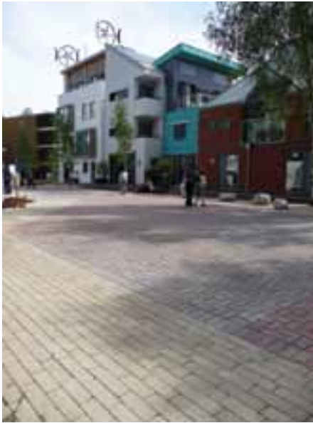
Concrete block permeable paving at the BRE Innovation Park.
