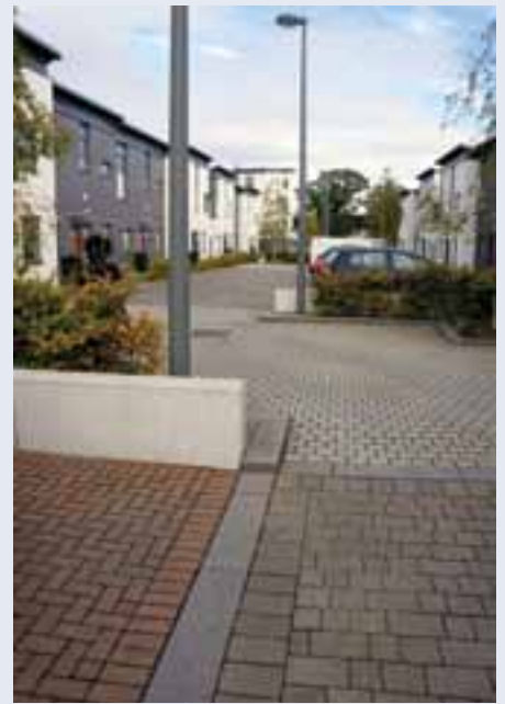
Permeable and conventional concrete block paving characterise these innovative, urban shared-spaces in Craigmillar, Edinburgh. Interpave case study available.
