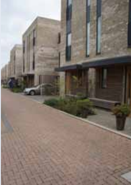
Permeable paving at Seven Acres (Skanska), Cambridge.
