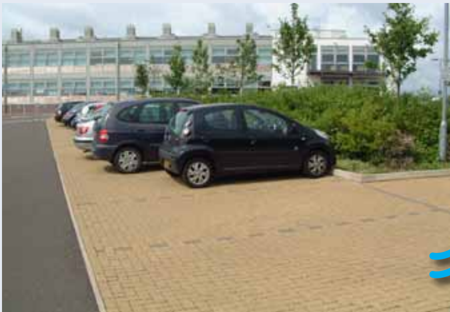
At the pioneering Hazeley School in Milton Keynes, a terraced sequence of permeable paving car parks provides effective pollutant removal for water serving two ponds for wildlife - notably the ‘protected’ great crested newts indigenous to the site. In addition, the ponds offer a valuable teaching and learning resource for the school.
