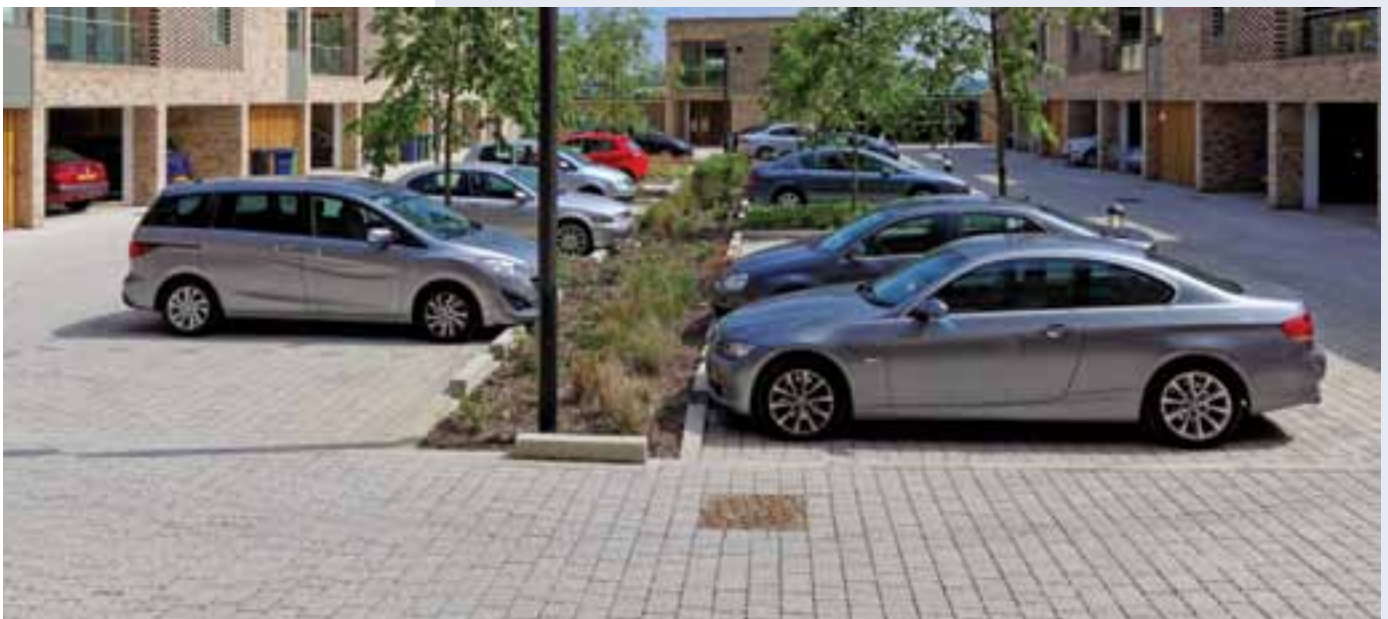
Permeable and conventional concrete block paving at the award winning 'Abode' housing, Cambridge. Photo: Simon Bunn (also front cover left hand image)
