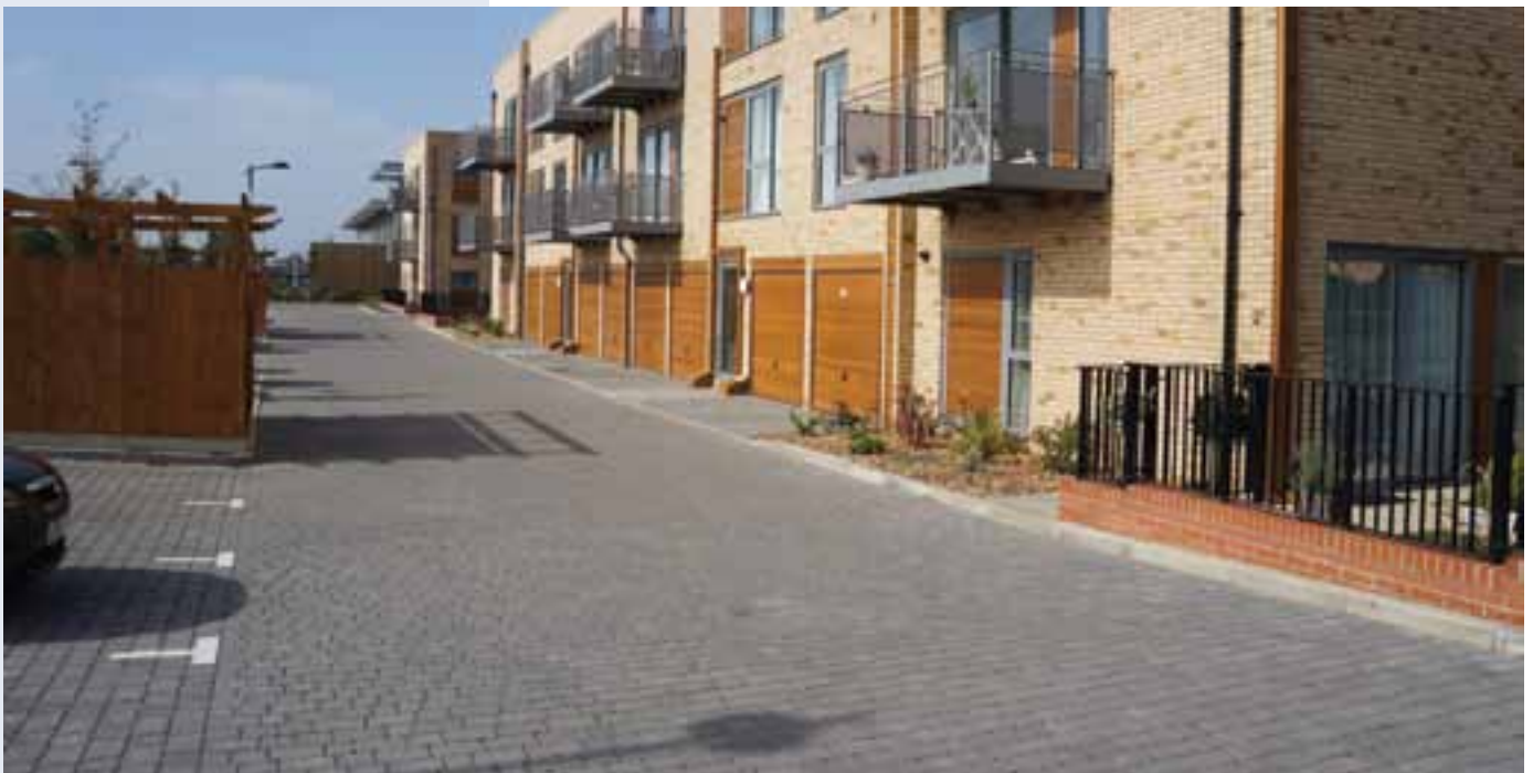
At Trumpington Meadows, Cambridge, concrete block permeable paving is used extensively. However, opportunities have been missed throughout the Cambridge developments in areas adopted by the local highway authority, dominated by impermeable surfaces and gulleys.
