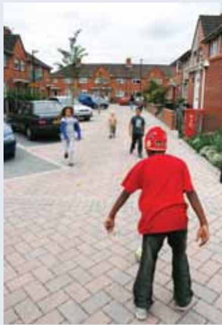
Retrofit concrete block permeable paving in Bristol.
