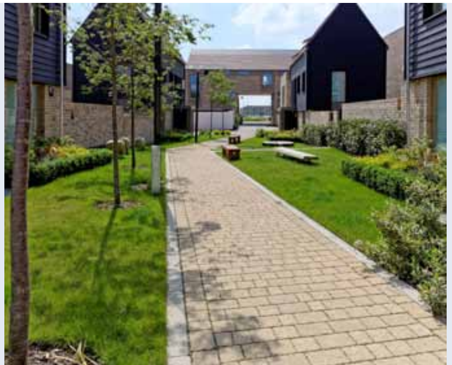
Pedestrian 'green lanes' in concrete block permeable paving traverse 'Abode', Cambridge. Photo: Simon Bunn.
