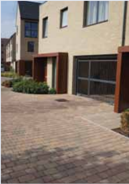
Permeable paving at Novo (Glebe Farm), Cambridge
