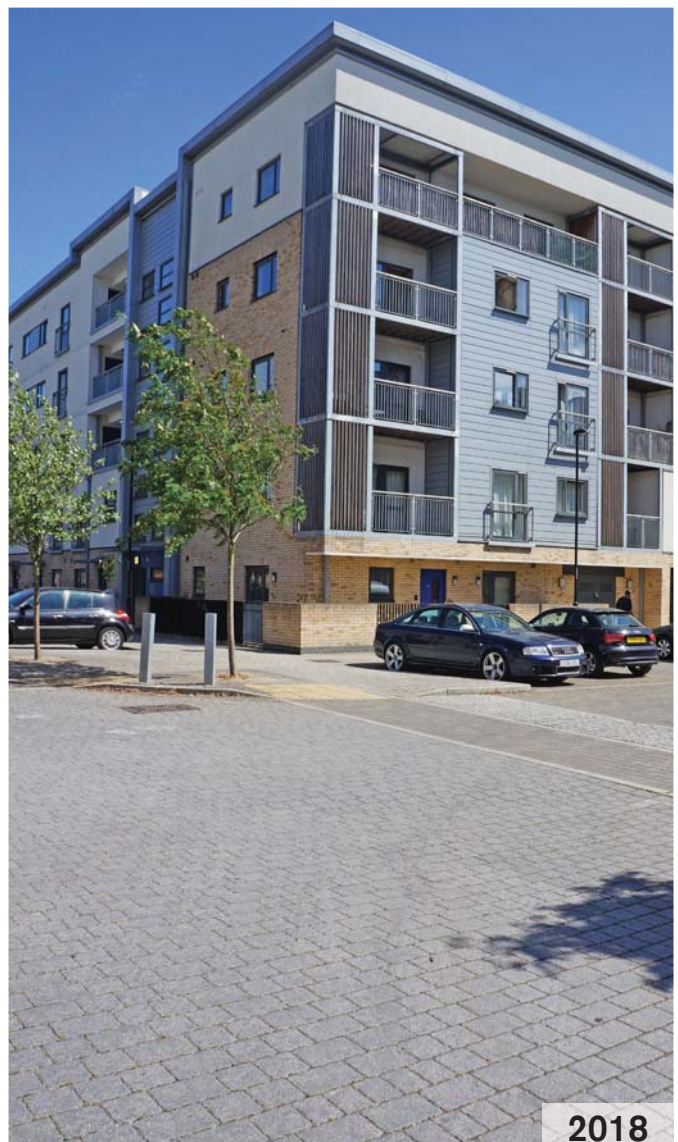
Phase 1 paving in 2018, as also shown on Page 5 some 6-years earlier.
