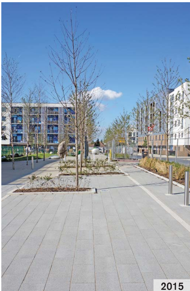
Local Square characterised by larger-format concrete block paving.
