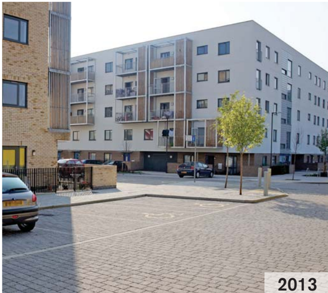
The Phase 2 Courtyard Block with concrete block permeable paving to the north.
