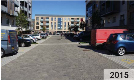
Phase 3 additions along the northern boundary, beyond Phases 1 and 2 concrete block permeable paving.
