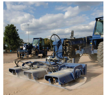
For even greater efficiency, machine-mounted jointing material spreading and (as shown here) compaction equipment can be used.
