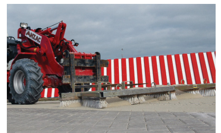
There is even machine-mounted equipment available for brushing in jointing material.
