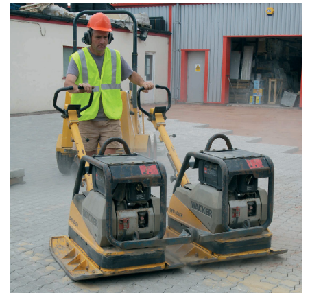
Banks of plate vibrators can be used for compaction.
