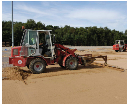
Machine based screeding equipment speeds up the laying course preparation.
