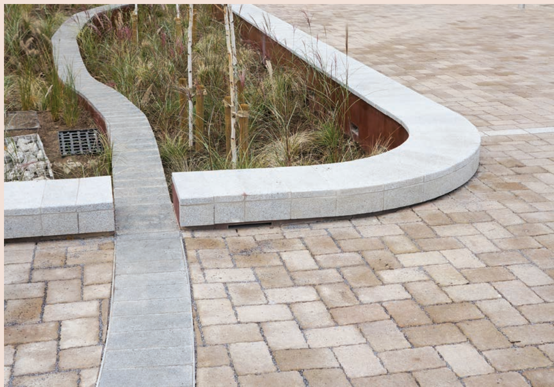
Water from the permeable paving simply discharges horizontally into the planted basins through slots in the side-walls.
