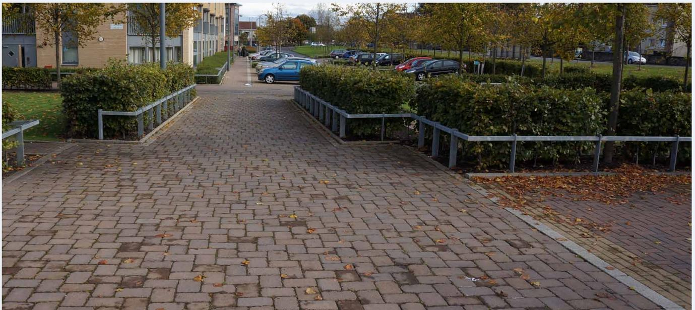
“Concrete block permeable paving is an ideal SuDS technique for high density housing, retaining a good quality finish with minimal maintenance.”
